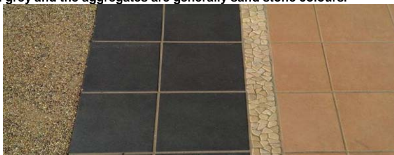
A photo of the paving used at the entry to Council showing the use of a range of earth colours plus the concept of a panel with a frame around.
