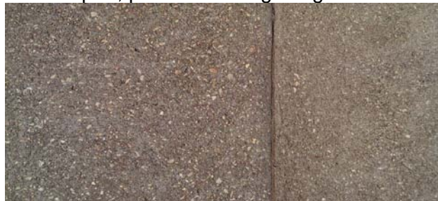
An example of a traditional footpath with exposed aggregate. The original colour of the cement in this case was standard grey and the aggregates are generally sand stone colours.
