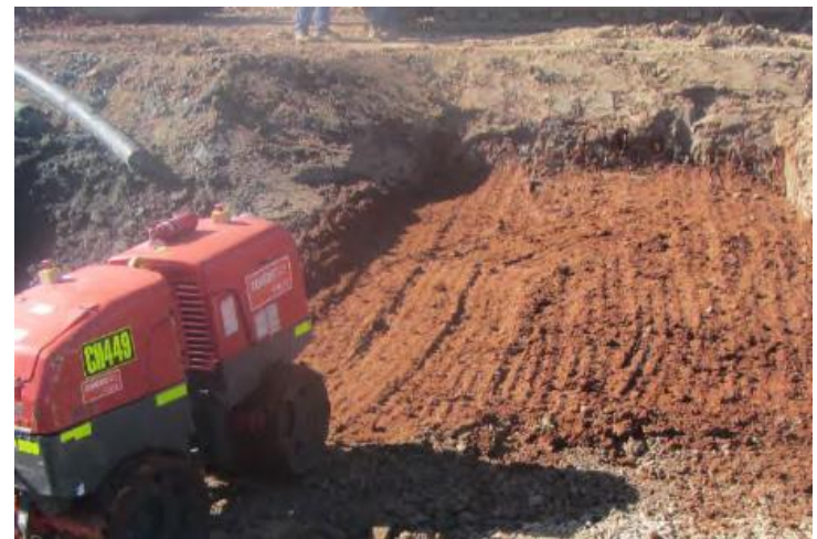
Example of reinstatement of clay liner (above and below)
