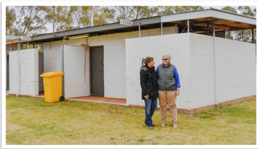
2018 Round 1 CPP – Weethalle Showground's Amenity Block Refurbishment
