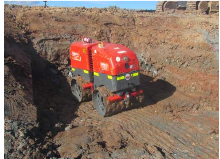
Example of reinstatement of clay liner (above and below)
