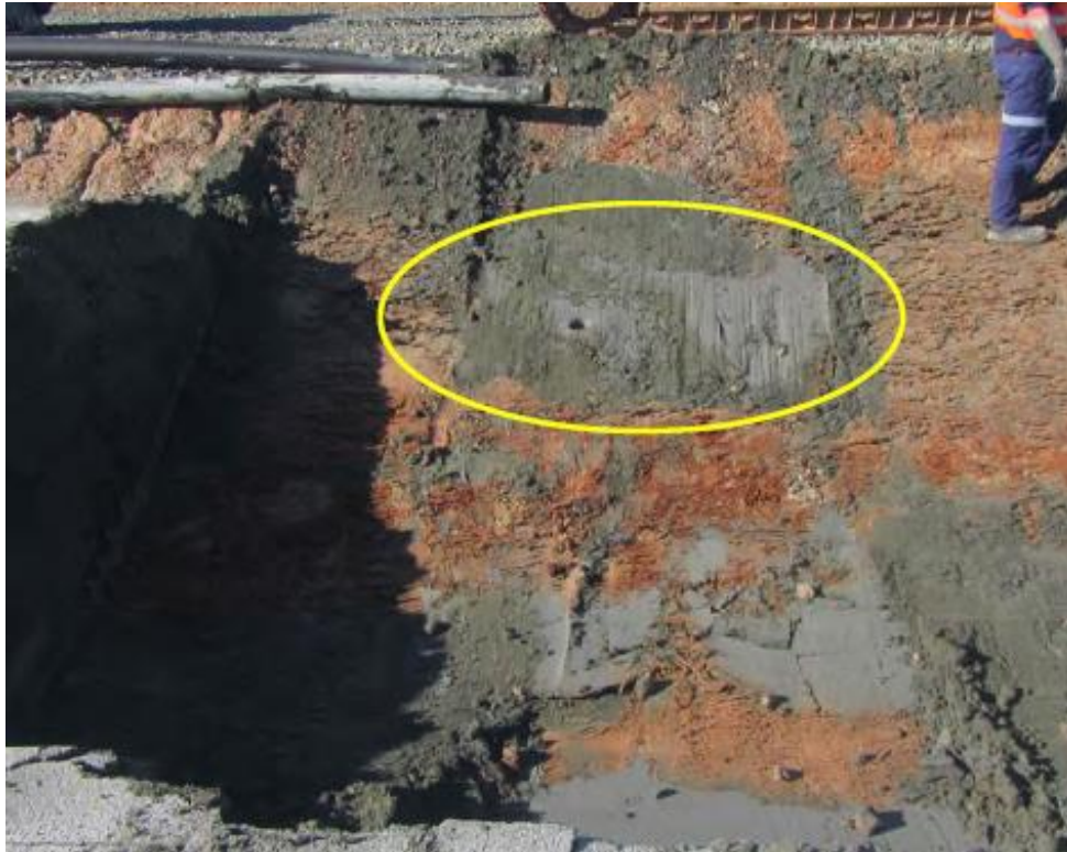
Clay liner with wet tailings exposed on eastern wall, Stage 5
