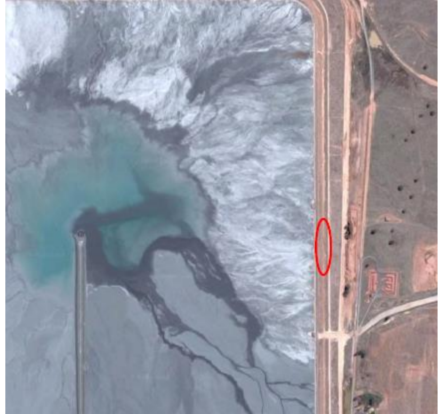
Approximate location of tailings breach (red oval)
