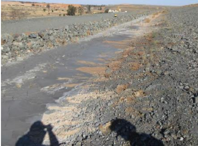
Tailings on Stage 4 NTSF berm, looking south
