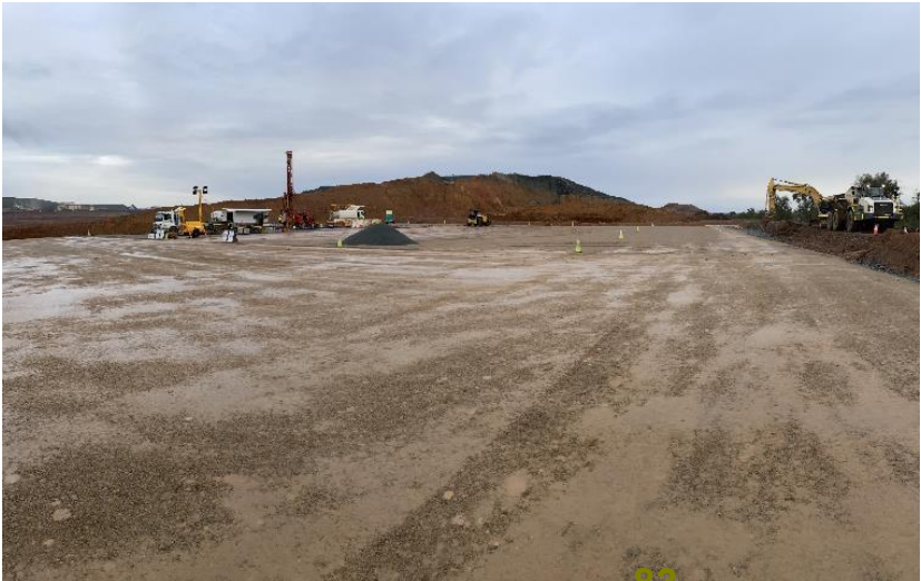
UG Paste Plant area preparation and vertical paste pilot hole drilling in preparation for larger rig in next stage of project
