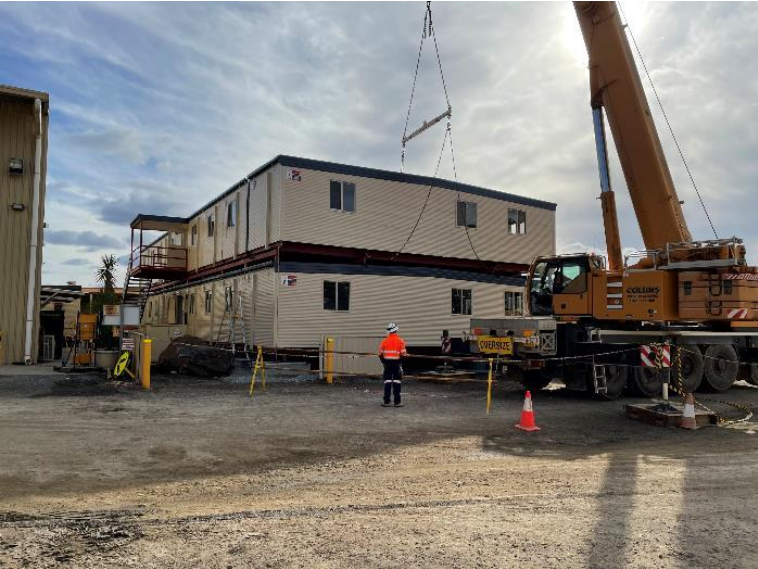
UG Admin buildings being installed
