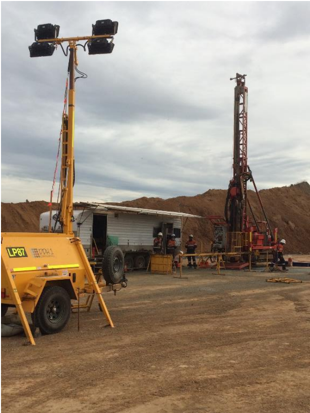
UG Paste Plant area preparation and vertical paste pilot hole drilling in preparation for larger rig in next stage of project
