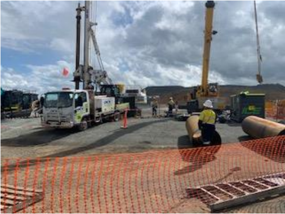
Piling contractor for silo area
