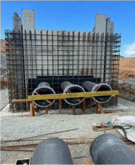
Service corridor catchment pit
