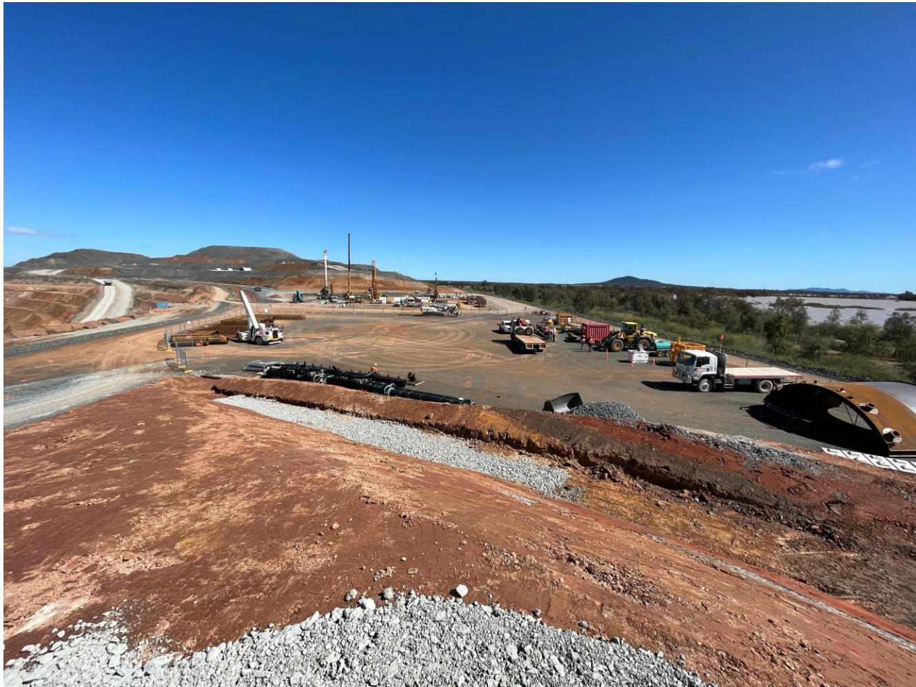
UG Paste Plant Precinct Construction Overview
