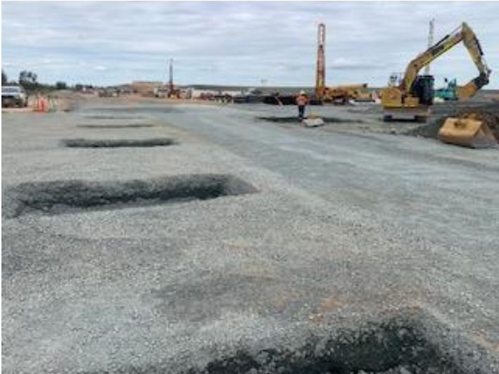
Services island foundation installation
