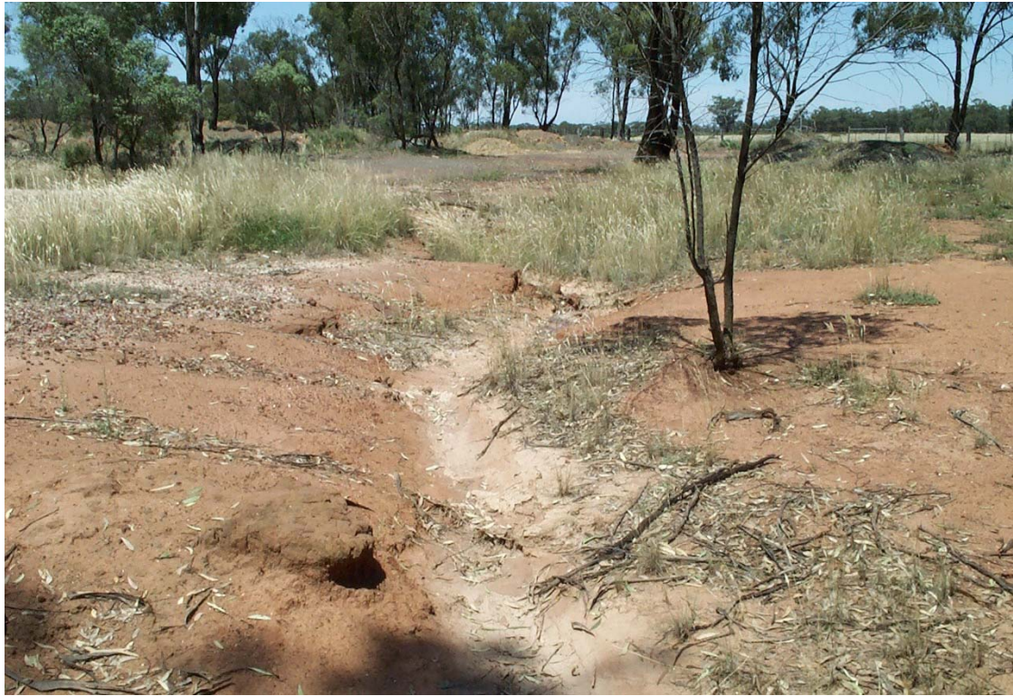
Photograph 7 Erosion at the West Wyalong Saleyards
