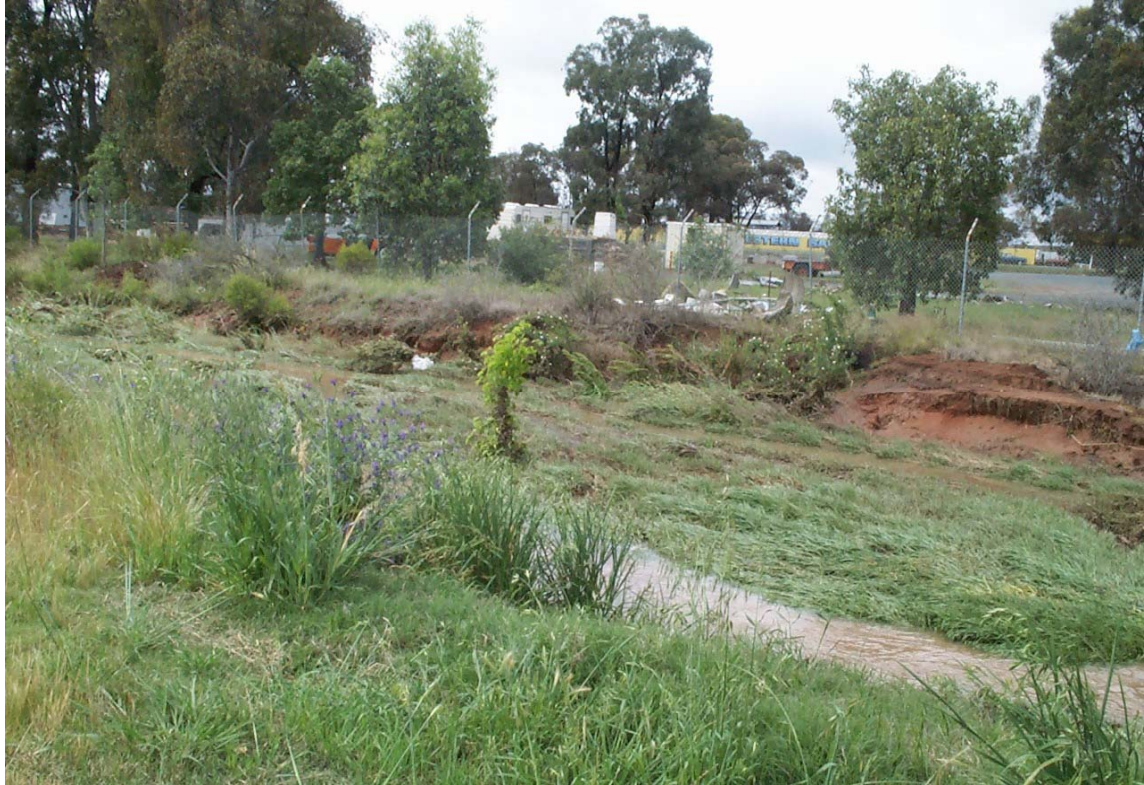
Photograph 3 Drains at Clear Ridge Road
