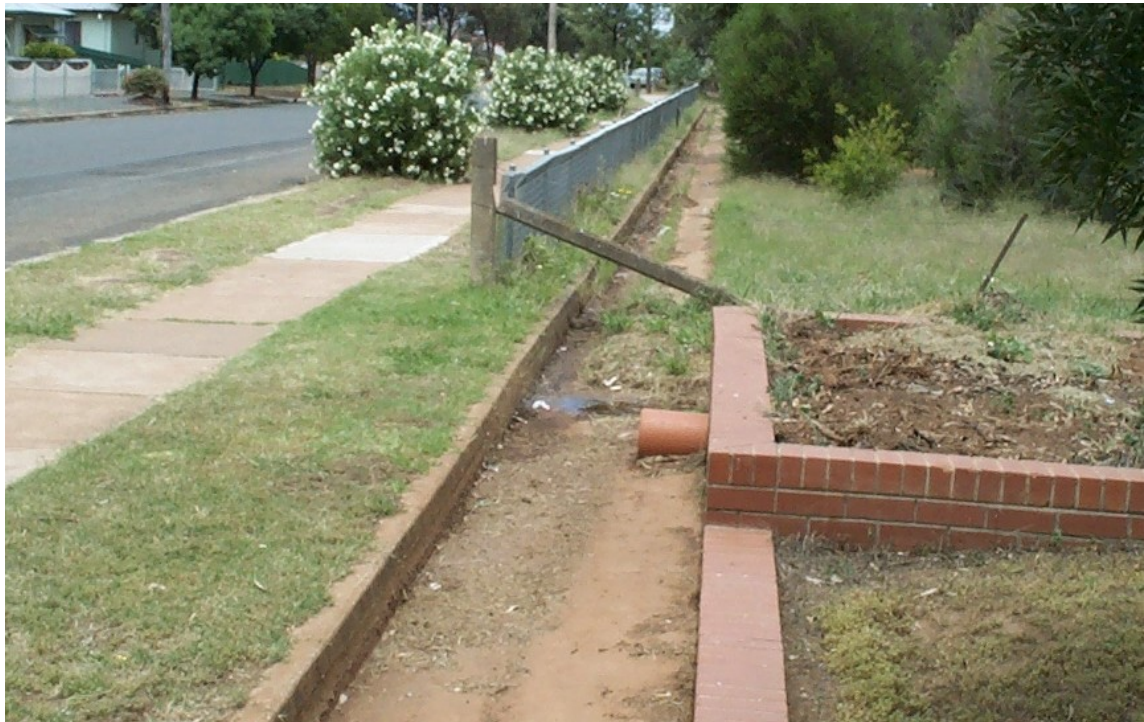
Photograph 4 West Wyalong High School
