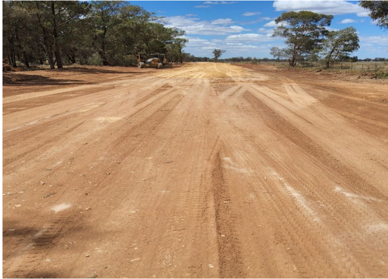
Figure 3 Road base being spread ready for compaction
