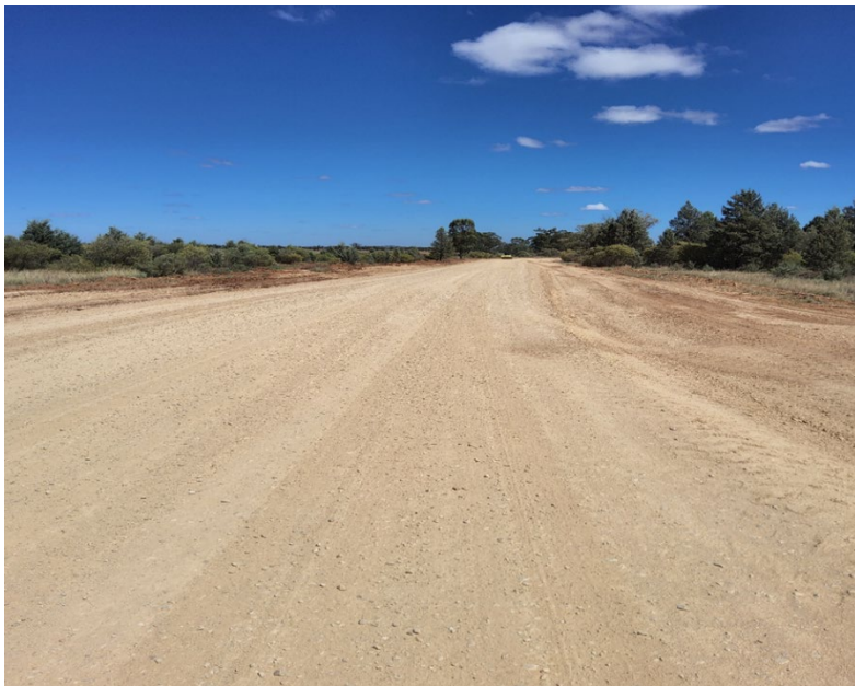
Figure 4 Road base installed, compacted and ready for final trim and sealing
