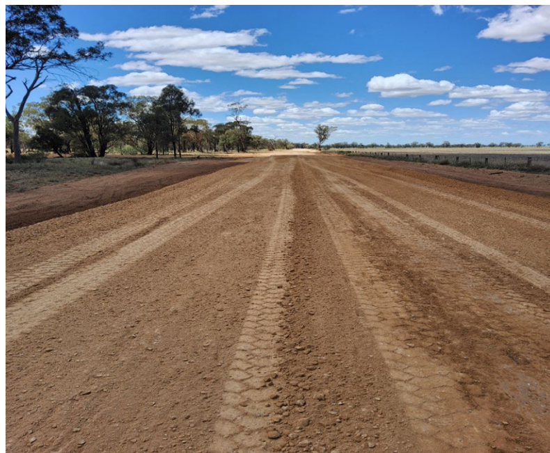
Figure 2 Road base installed and ready for compaction
