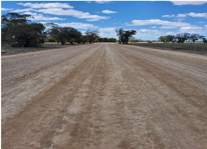
Figure 1 Road Base installed ready for compaction
